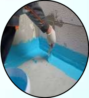
Building renovations/Seepage /Water Proofing
